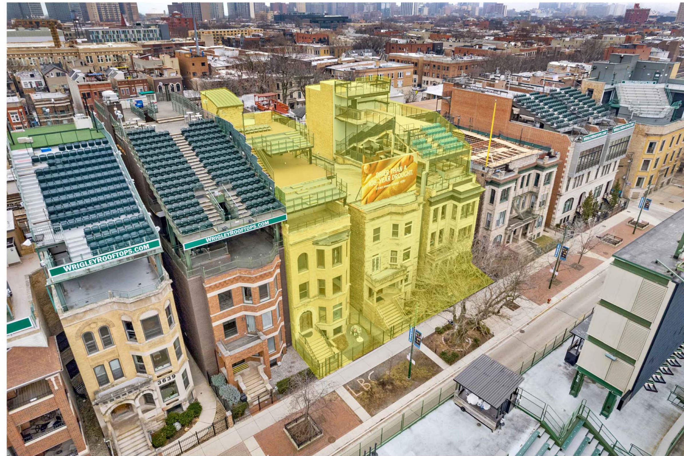
1: AERIAL OF EXISTING BUILDINGS, LOOKING SOUTH-EAST
