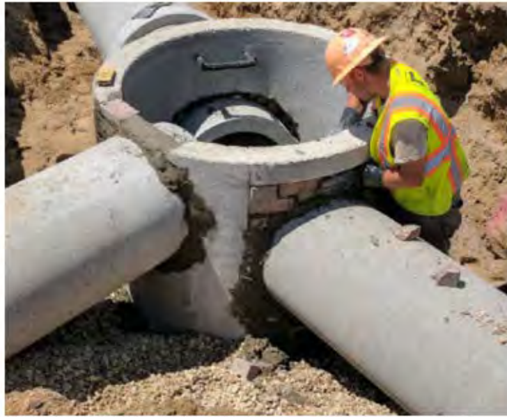
PROPOSED DRAINAGE STRUCTURES AND PIPES (I.E. STORM SEWER, CATCH BASIN, CONNECTION TO EXISTING DRAINAGE, ETC.)
