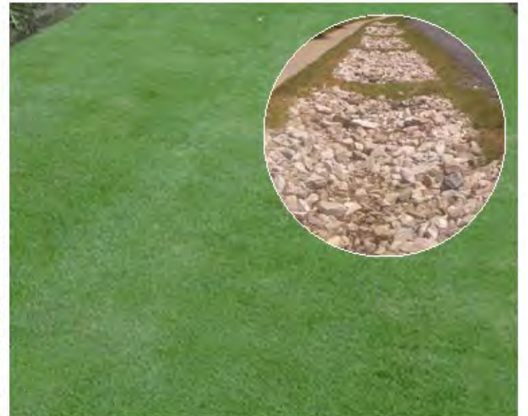
INFILTRATION TRENCH (I.E. LINEAR CHANNEL WITH SPECIFIC SLOPE, HARDSCAPE MATERIAL AND PLANTING MATERIAL, ETC.)
