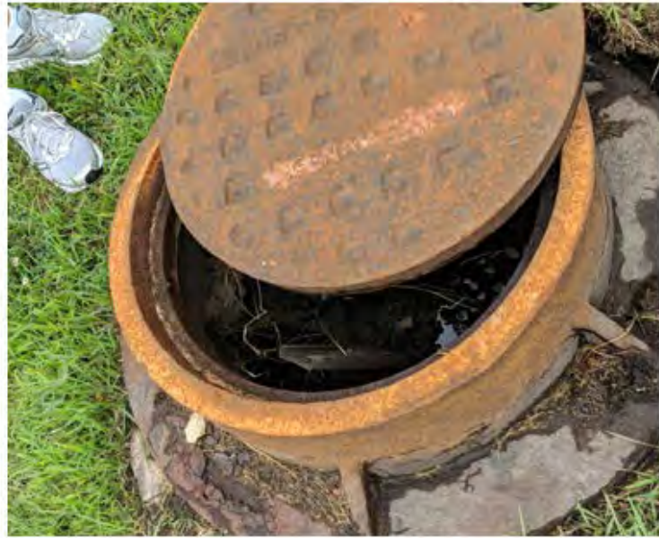
PRESERVE AND CLEAN EXISTING DRAINAGE STRUCTURES ON-SITE
