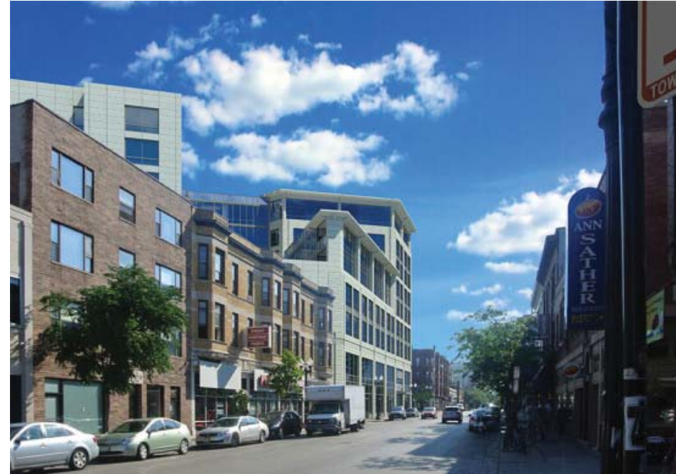
VIEW EAST DOWN BELMONT
