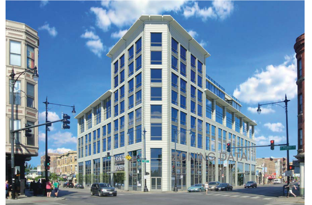
PROJECT TO BE COMPLETED AT INTERSECTION OF CLARK AND BELMONT
