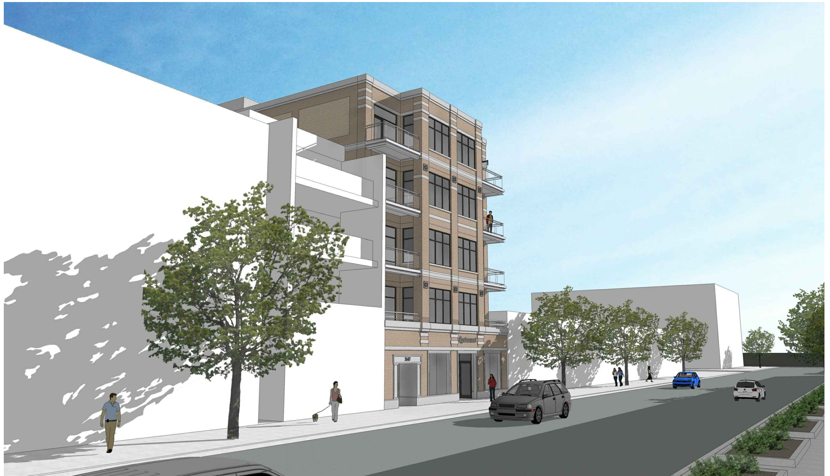
VIEW ALONG N. SOUTHPORT LOOKING SOUTHEAST
